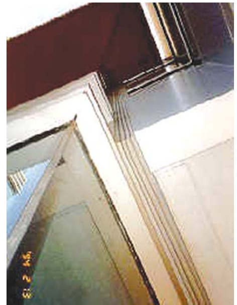
Unique among options for large joint-gap sealing, COLORSEAL an SEISMIC COLORSEAL can be positively secured at inside corners without invasive anchors. In addition the products' ability to maintain watertightness while handling curves and directions changes further sets it apart from rubber-and-rail strip seals.
