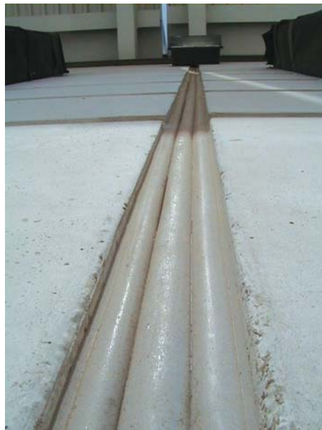
Unique among options for large joint-gap sealing, COLORSEAL an SEISMIC COLORSEAL can be positively secured at inside corners without invasive anchors. In addition the products' ability to maintain watertightness while handling curves and directions changes further sets it apart from rubber-and-rail strip seals.
