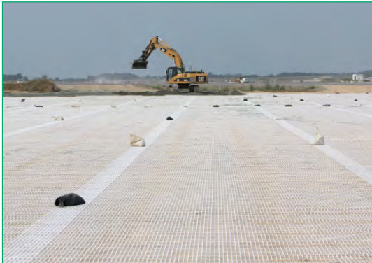
Fig. 7 Installed Secugrid® as a base course reinforcement
