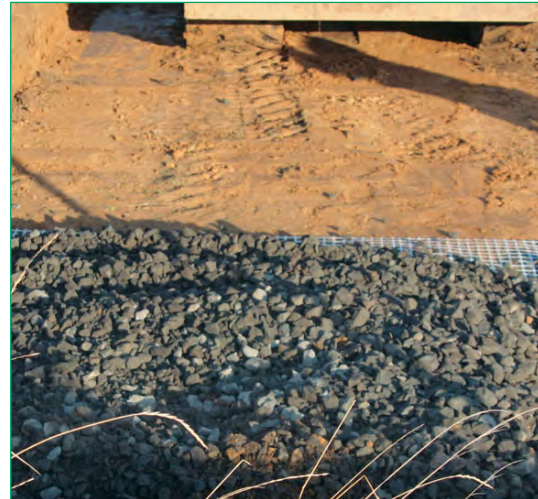
Fig. 17 Placement of base course gravel over the Secugrid® section
