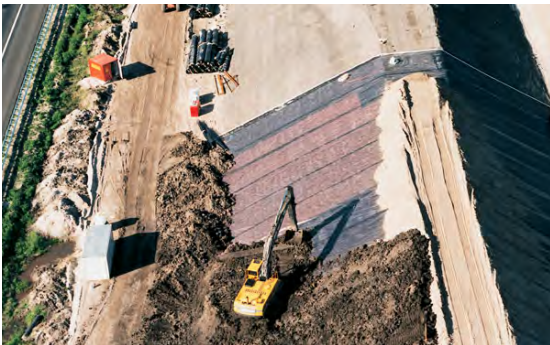
Slope reinforcement of a noise barrier with Secugrid®
