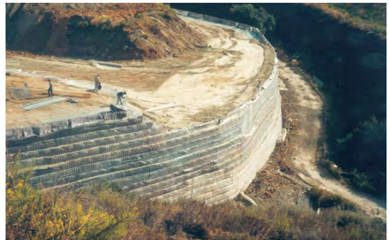
Mechanically stabilised earth (MSE) wall construction
