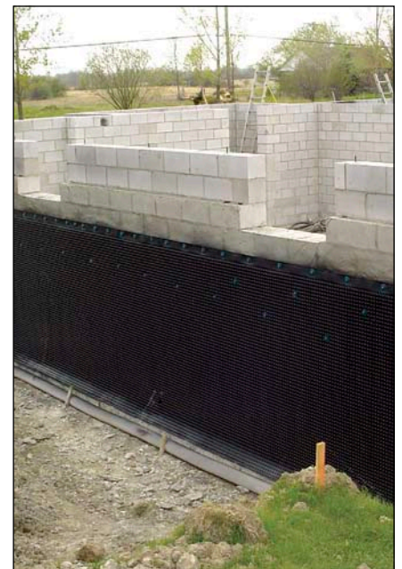
DMX FlexSheet™ applied to foundation wall eliminates the effects of Capillary Suction and Hydrostatic Load.
