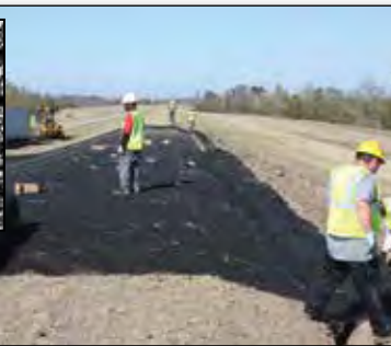
US Army Corps of Engineers Levee Construction
