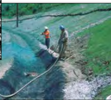
Slope interceptor ditch on steep slopes
