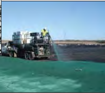
Flexterra® HP-FGM™ applied into TRM 7003
